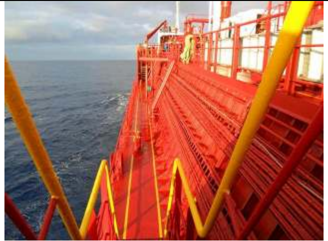
12. MAIN DECK FWD PORT
